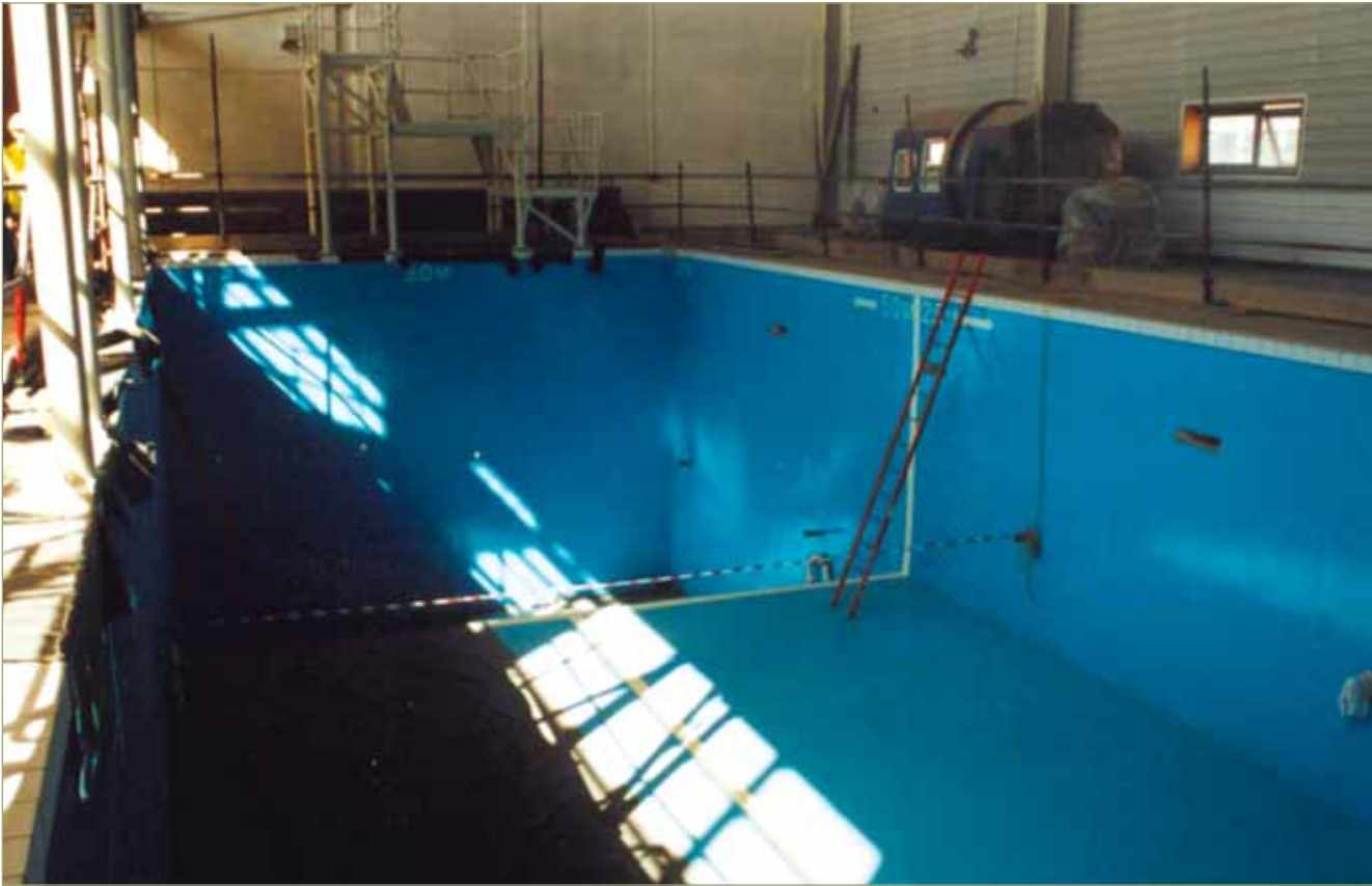
The impressive dive pool under construction at the National Maritime College.
